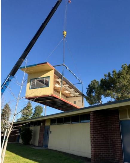
**Photo 5: A crane moves a new portable building into place on Shull Elementary School's campus to accommodate increasing enrollment.**
